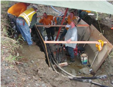
Tropical conditions including torrential rains punctuated by Cyclone Larry made this job hot and wet. Injection adaptors to accommodate the large conductor and thick insulation were easy to install. Conductor compression ranged from round to compressed to compact. Each cable subsegment was provided with a customized formulation tailored to its strand compression.
